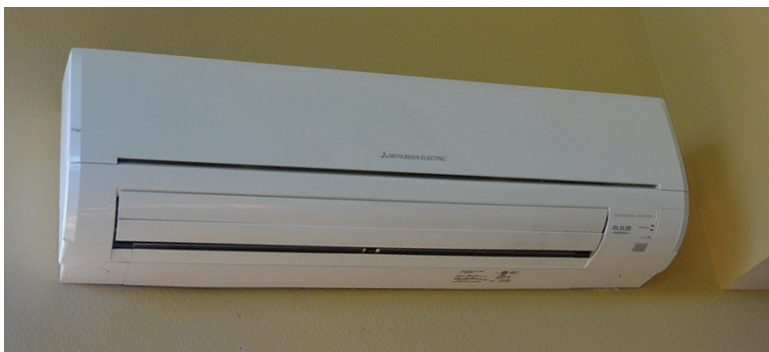
heat pump system—inside photo by Pat Welle
