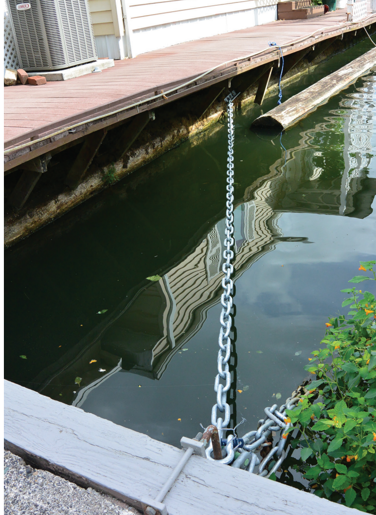
mooring connection of galvanized chains photo by Pat Welle
