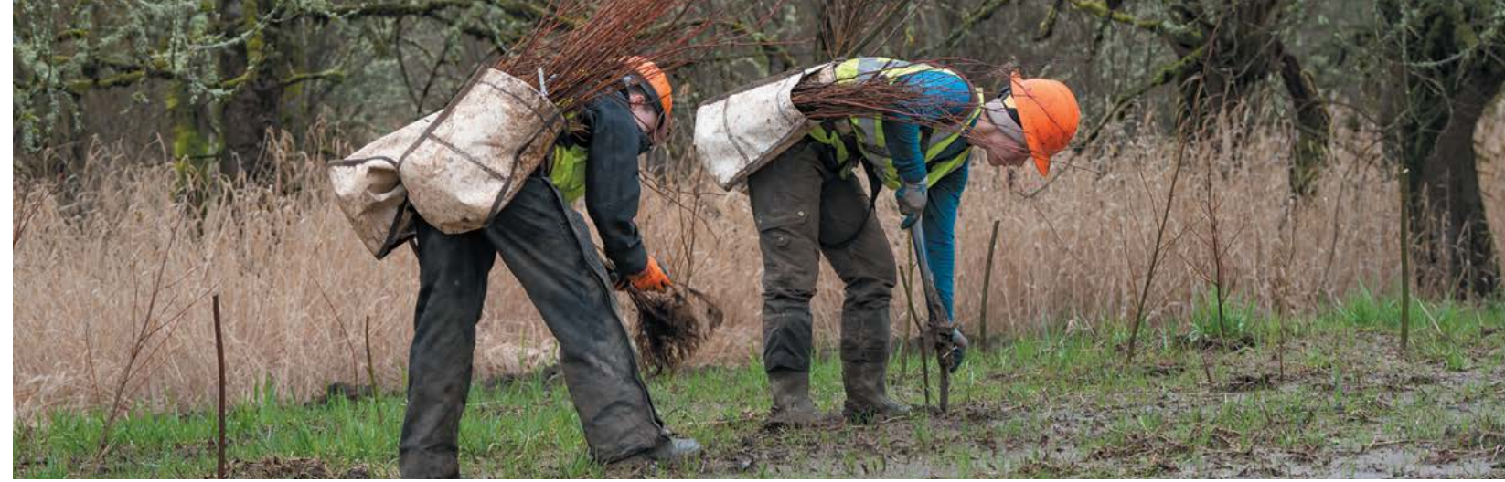
Crews plant willow on a wetland restoration site. Photo by Pat Welle.
