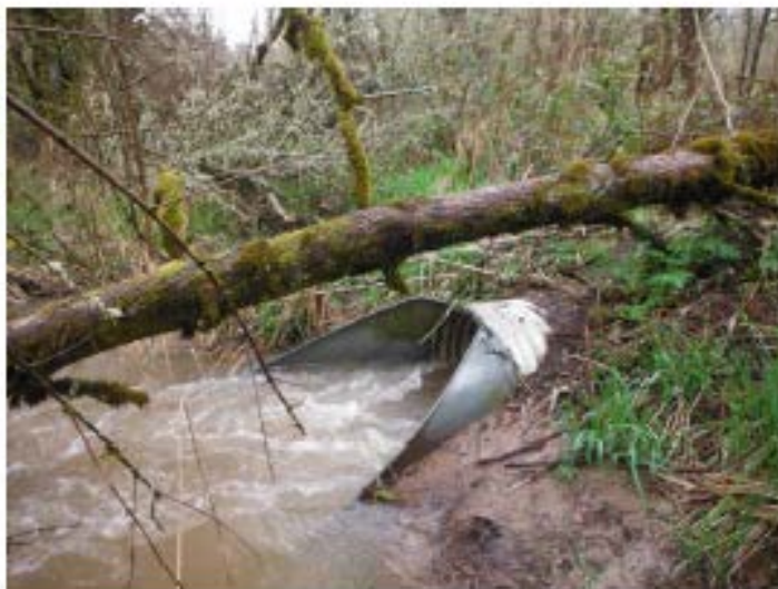
Culvert to be replaced with channel spanning bridge
