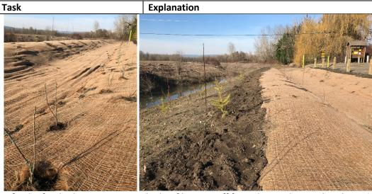
**Left:** The finished stormwater swale that filters runoff from the Reeder Road Bridge. **Right:** the swale and some of the plantings along the banks of Dairy Creek.
