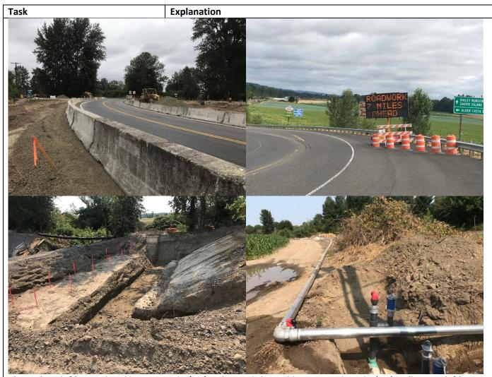
**Photo:** (Top left) Completed bypass road 7/18/18, (top right) variable message board 7/19/18, (bottom left) excavated southern bridge footing 7/30/18), (bottom right) some of the pipe work to keep the farmer's irrigation working through construction 7/30/18.
