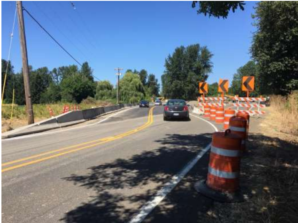
Opening of bypass roadway
