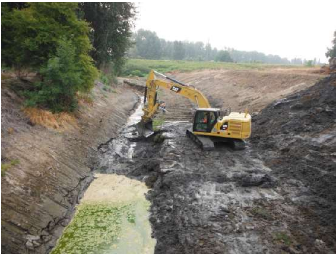
Very soggy working conditions
