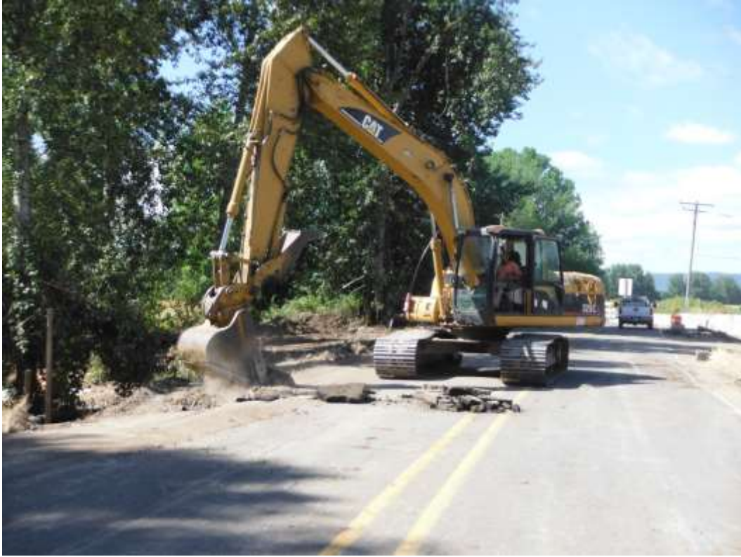
Tearing up old roadway
