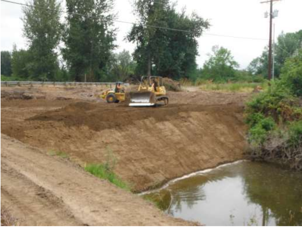
Construction of bypass roadway
