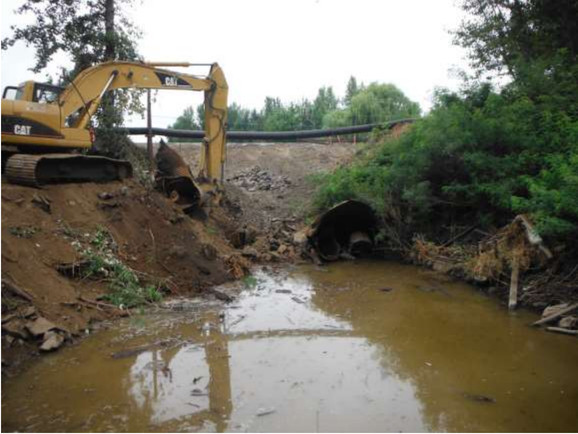
Removing portions of the old culverts
