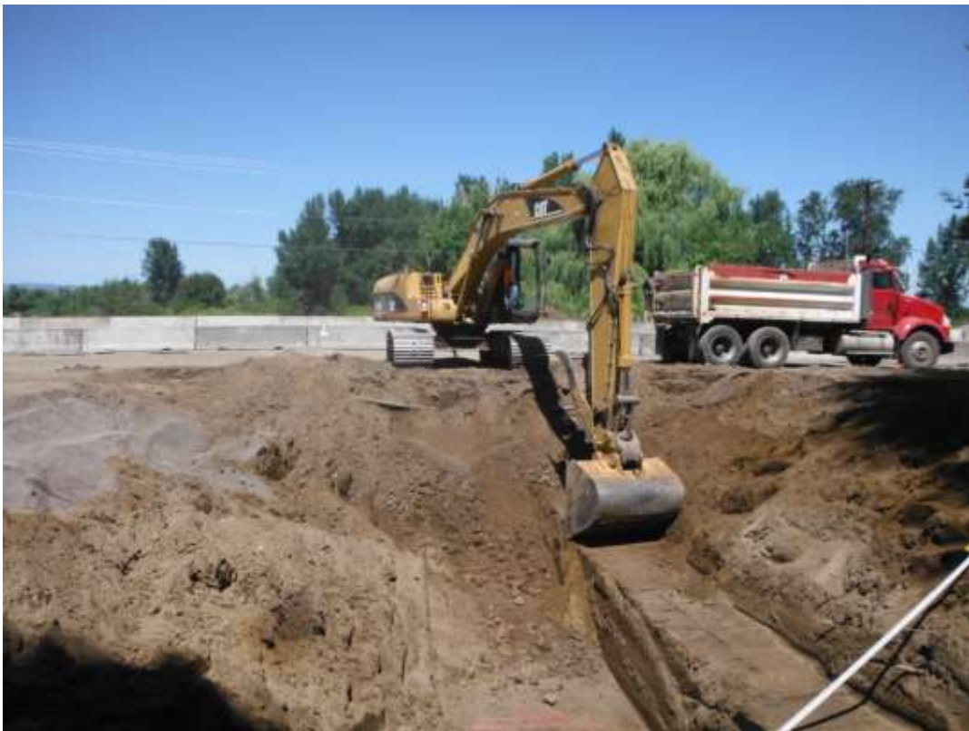
Excavating bridge abutment footprints
