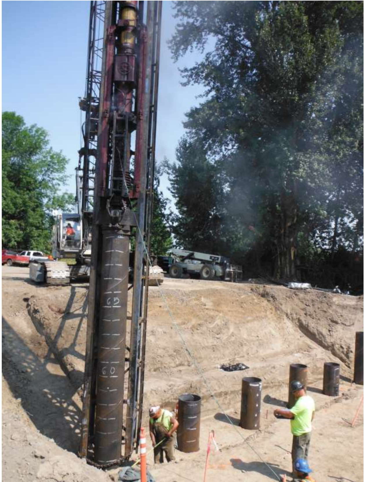
Driving piles for the bridge
