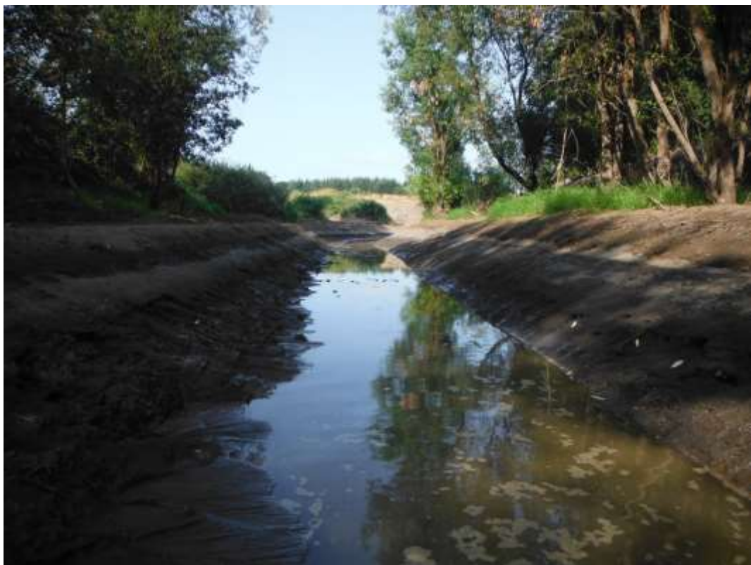
Channel being cut through old debris plug (August 22, 2018)
