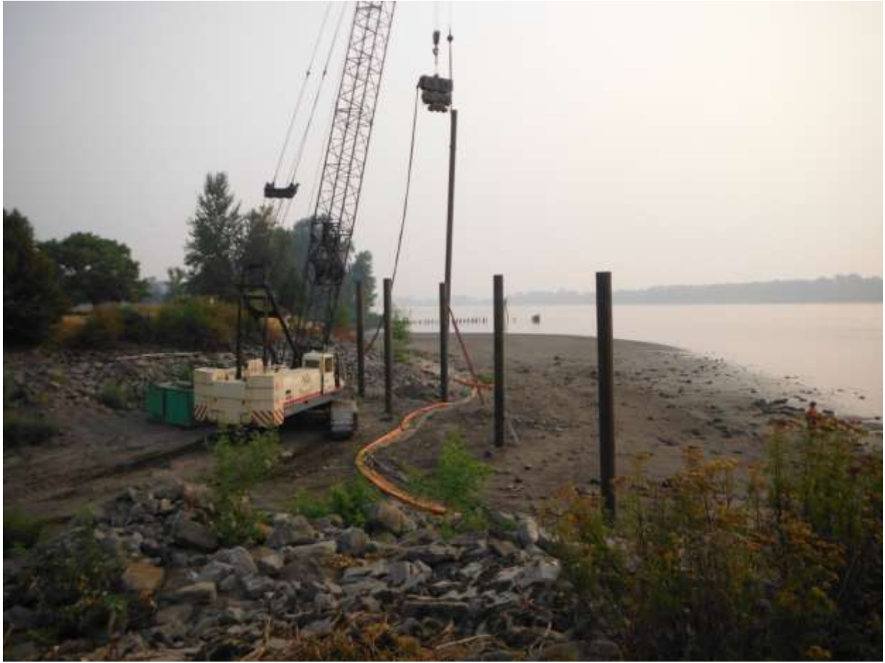
Installing debris boom pilings
