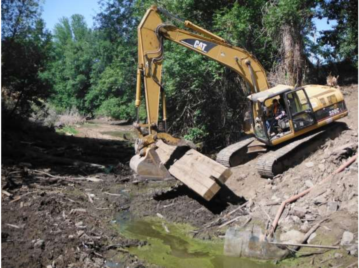
Beginning the channel work
