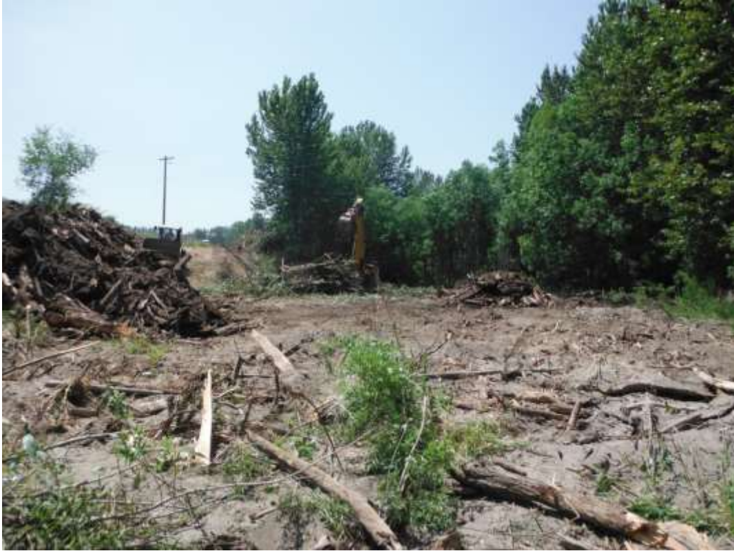
Removal of debris plug
