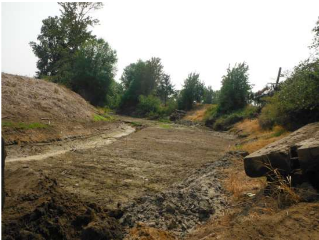
Channel and marshplain bench taking shape (August 10, 2018)
