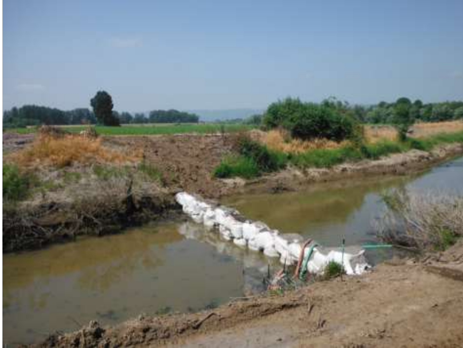
Installation of sandbag cofferdam
