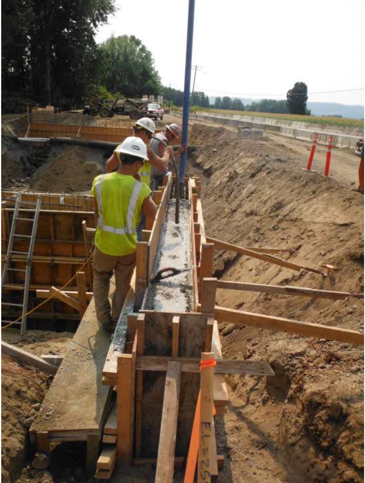
Pouring concrete for northern abutment and wingwalls
