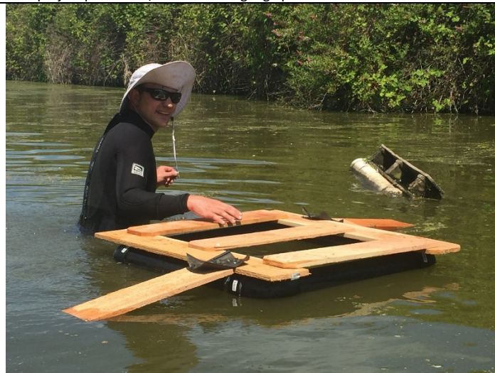
New turtle basking rafts being installed on Sauvie Island canals
