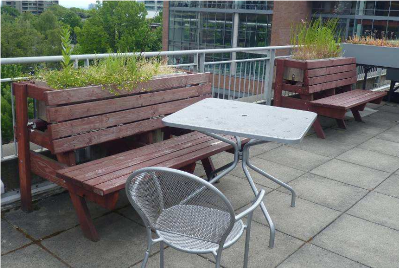
Figure 2 These benches were created to intercept some rainfall and seat people on a roof terrace.
