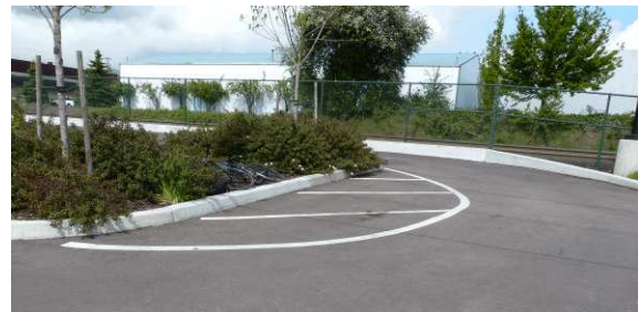
Figure 1 Many small unused pavement areas add up to a lot of unnecessary pavement in a watershed.
