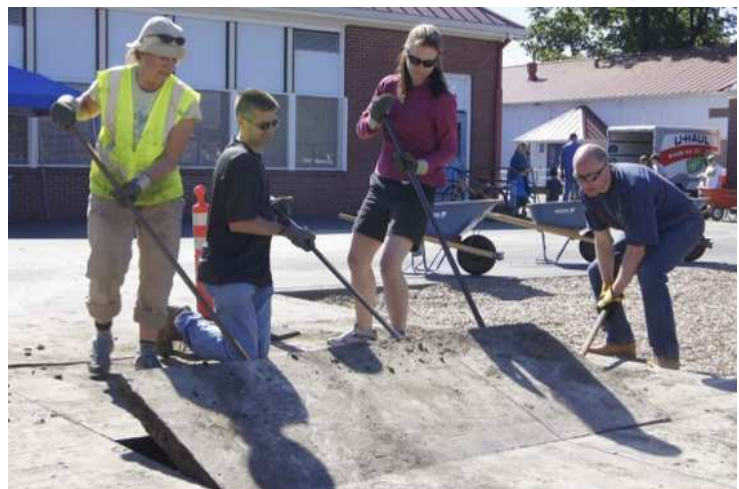
Figure 3 Volunteers learn about the connection between impervious pavement and water quality as they work to remove asphalt at a school.
