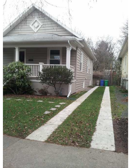
Figure 1 Homeowners often don't use the entire paved area of their driveway. In Portland, this driveway configuration reduces runoff by about 5000 gallons/year.
