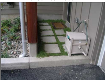
Poured in place permeable pavers ($$)
