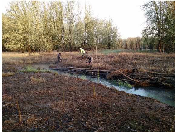
Photo: Restoration crews installing willow cuttings along McCarthy Creek in early 2018 (Credit: WMSWCD)
