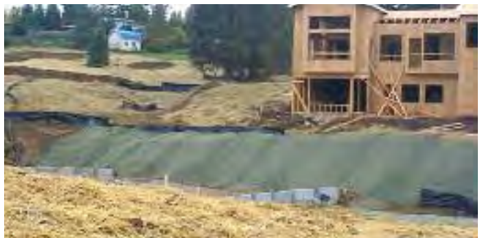
straw mulch used to prevent erosion
